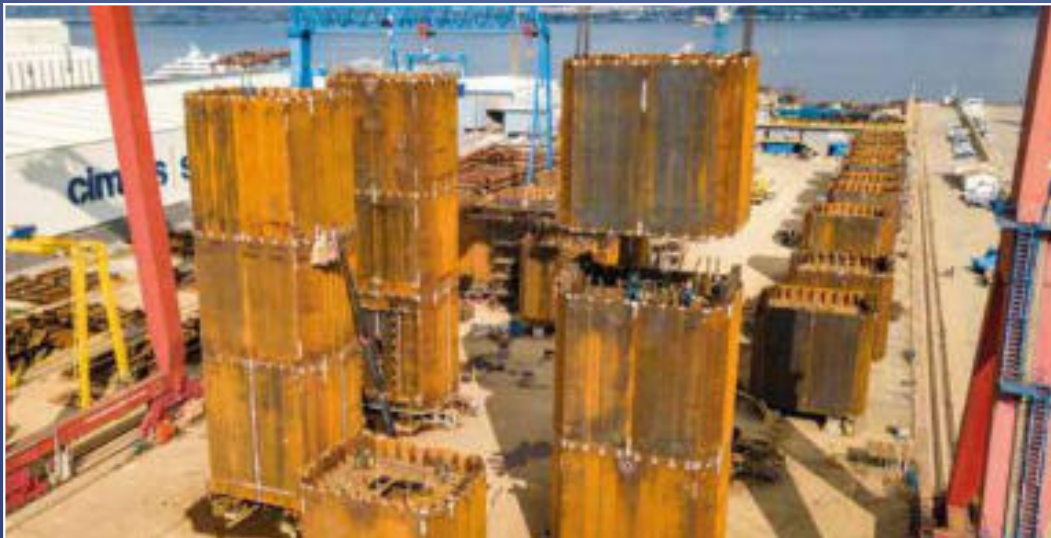
TOWER BLOCK TRIAL ASSEMBLY
