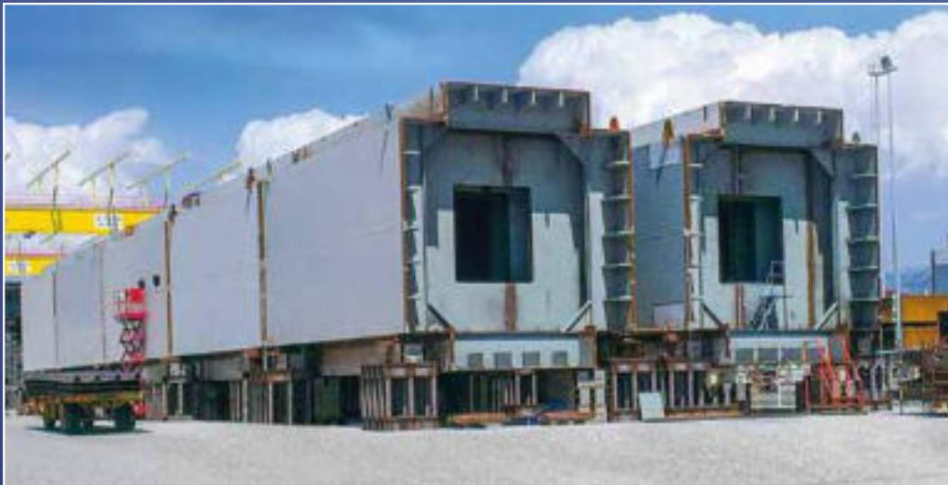
TOWER BLOCK TRIAL ASSEMBLY
