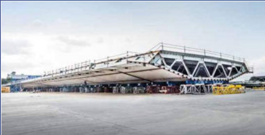
GIRDER BLOCK TRIAL ASSEMBLY
