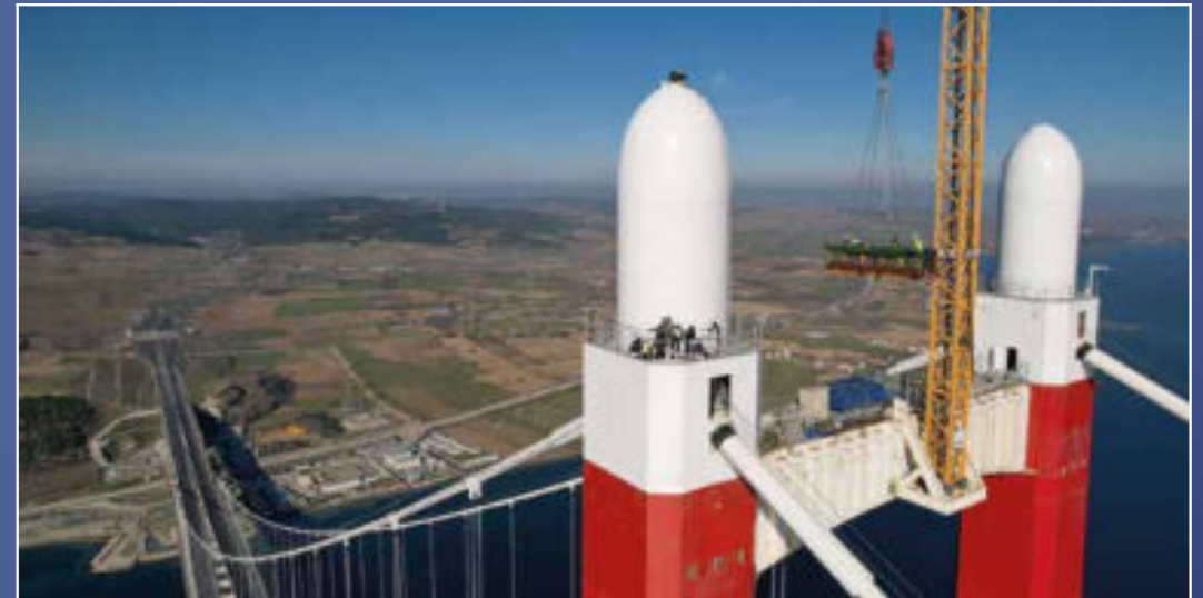
TOWER TOP ENCLOSURE INSTALLED
